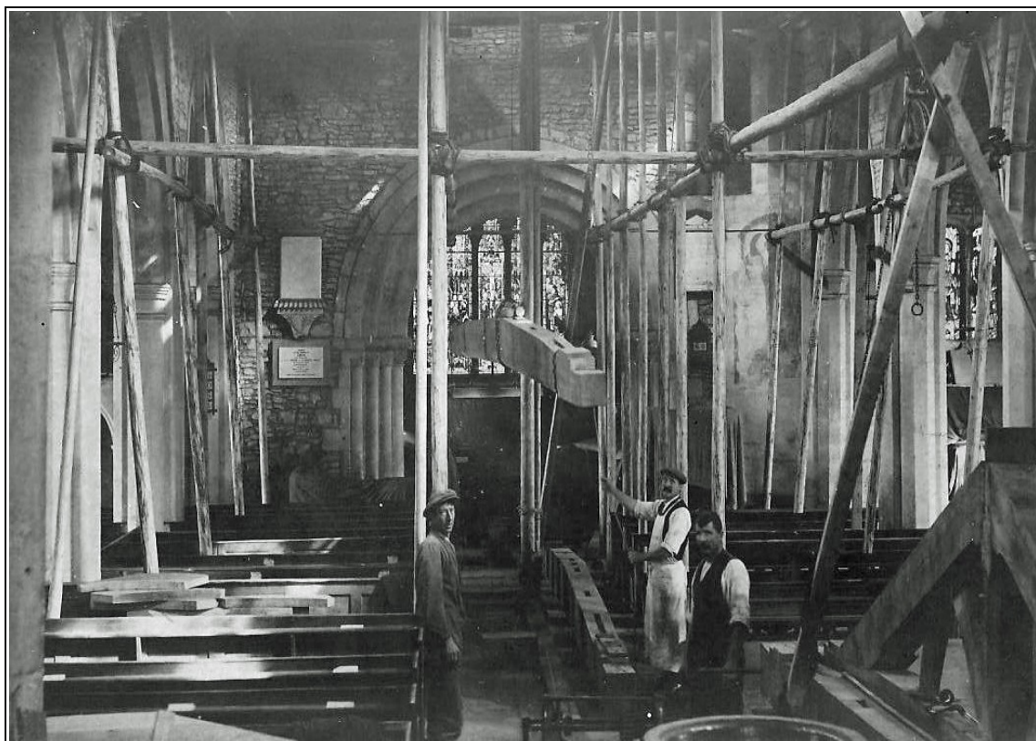
The nave during 1904-5 repairs
