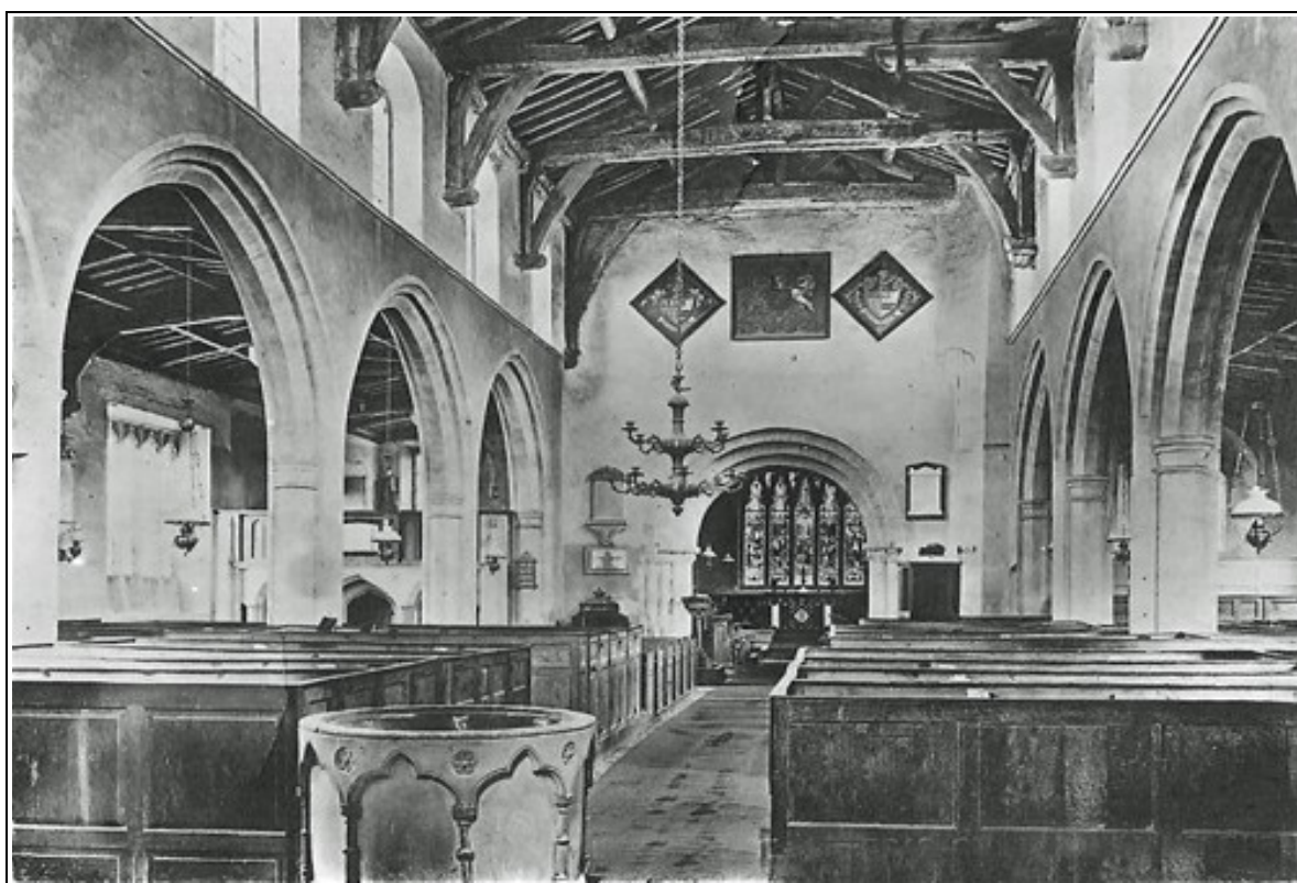
The nave before 1904
